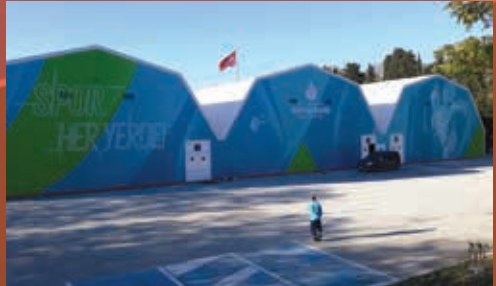
FLORYA TENNIS HALL Year of Construction : 2016 Size / Material : 3x18Mx36M PVC Membrane Frame : S350 Grade Light Steel Frame Location : Istanbul / TURKEY
